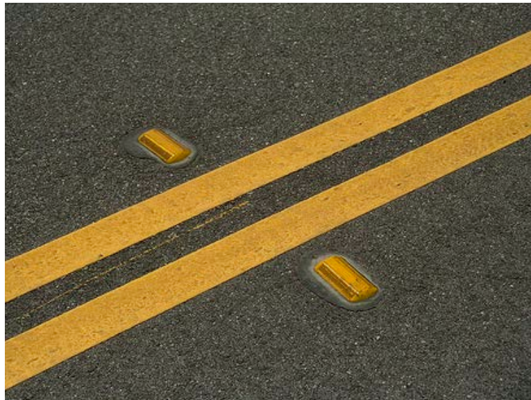
Pavement markings and reflectors
