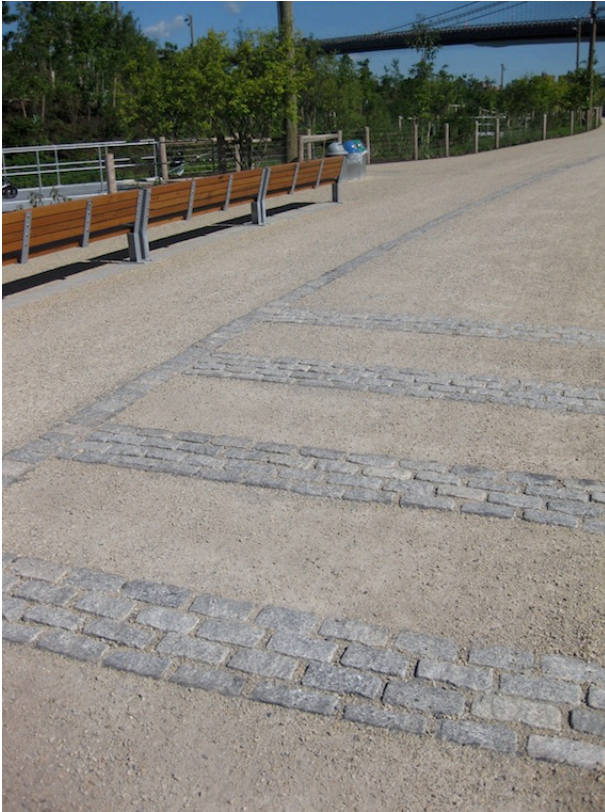
In-grade textured surfacing
